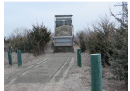
Construction on the Redbud Trail in Andover
